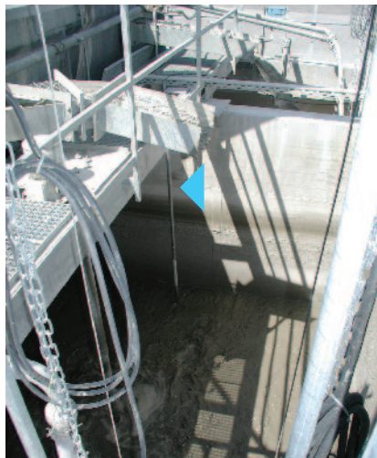
Installation CUS41/Sensor in the basin
