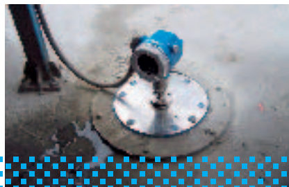
Level measurement with Micropilot M radar measuring system
