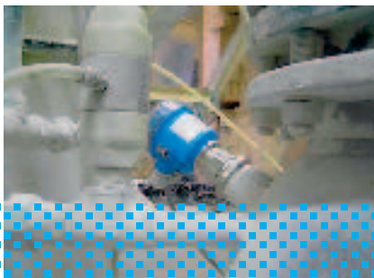
Limit detection in pneumatic pressure vessel with Soliphant M
